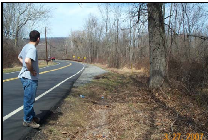
Open area near SDO-186 Ditch discharge
