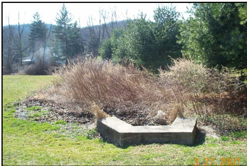
Vegetated stormwater discharge
