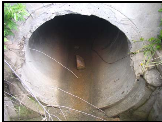
Inside pipe of outlet structure
