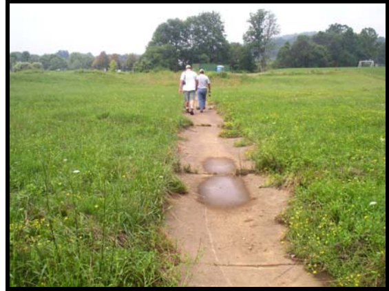
Low flow channel looking away from outlet
