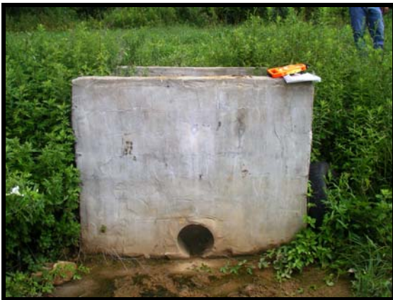
Outside orifice of outlet structure
