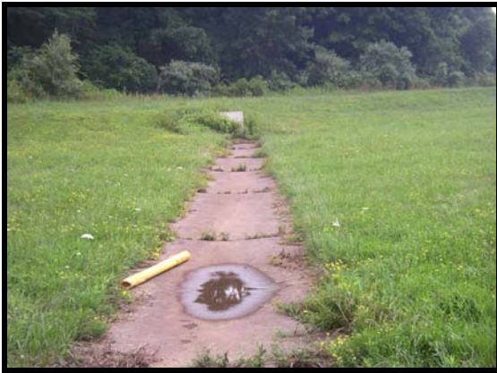
Low flow channel looking towards outlet
