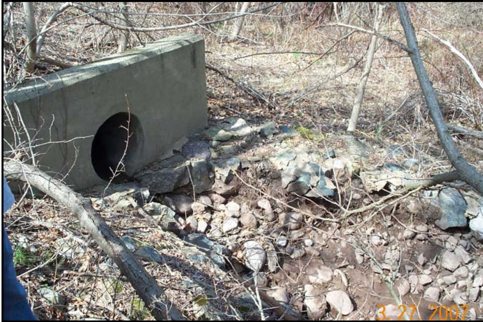
Stormwater outfall
