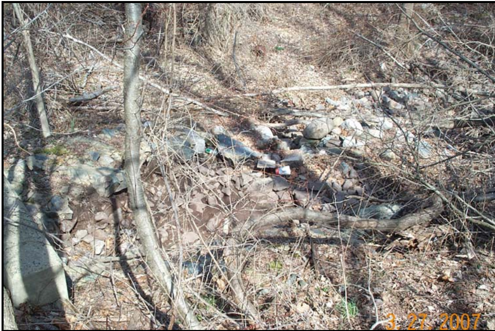
Sediment and trash deposition
