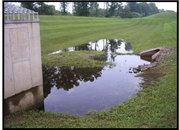
PV2 outlet and inlet (note close proximity)
