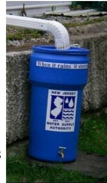
A rain barrel collects water from a downspout.
