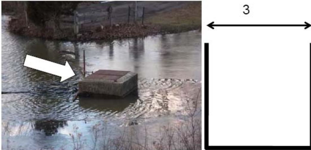
Figure 26. Golf Course Pond - Existing Outlet Structure
